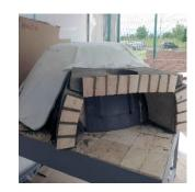
**Step 5**: Assemble the arch section as shown with one arch firebrick as the base each side. You can stick on slip bricks now or towards the end.
