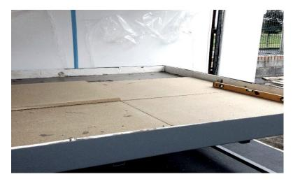
**Step 2**: Put down a layer of vermiculite board.
