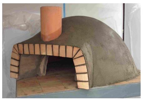
Step 10: If the oven is outside the vermiculite concrete must be covered with a thin layer on concrete or some other protection. Leave to set for at least 24 hours. Then dry slowly in open air or with small fires.
