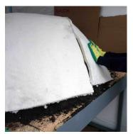
**Step 6**: Cut & stick the fibre blanket to the dome using Dinset / Cement.
