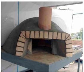
Step 8: A second layer of blanket and 4" / 100mm layer of Vermiculite cement may be added to the top of the dome to ensure no heat loss. Insert flue in chimney opening. Use Dinset to secure.
