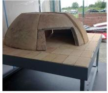
**Step 3:** Place the oven floor sections in position. Fix in place using a thin layer of Dinset. Place the dome, without mortar, in position.
