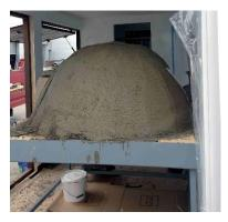
**Step 7**: Cover dome with 4" / 100mm Vermiculite concrete.
