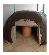
Insert the door to make sure it fits correctly before jointing the pieces. If there are any larges gaps between dome pieces mix Dinset with fibre blanket and fill the gap.
