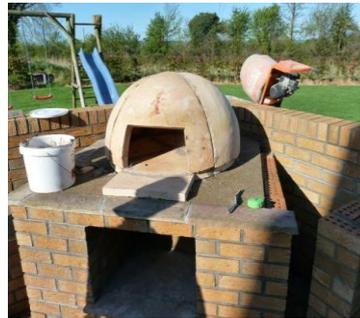
**Step 4:** Place the oven floor sections in position, centred on the base. Fix in place using a little cement / Dinset. Place the dome without mortar in position.
