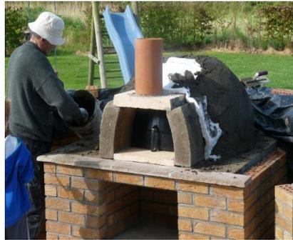
**Step 8:** Cover dome with 4" / 100mm vermiculite. A second layer of blanket and cement may be added to the top of the dome to ensure no heat loss.
