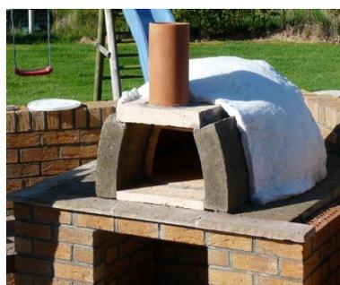
**Step 7:** Cut & stick the fibre blanket to the dome using Dinset / Cement.
