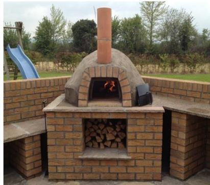
**Step 9:** Stick on slip bricks and add second flue if required.
