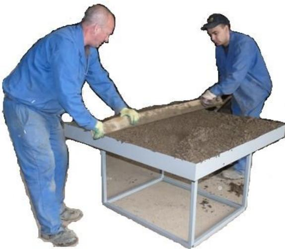
**Step 2:** Put down a layer of 25mm fibre blanket. On top of this form a 4" / 100mm layer of Vermiculite Concrete.
