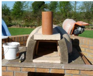
**Step 6:** Put on top flue gather brick and insert flue in chimney opening. Use Dinset to secure.
