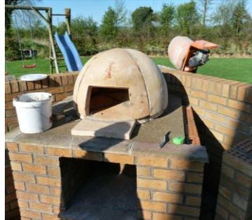
**Step 4:** Place the oven floor sections in position, centred on the base. Fix in place using a little cement / Dinset. Place the dome without mortar in position.
