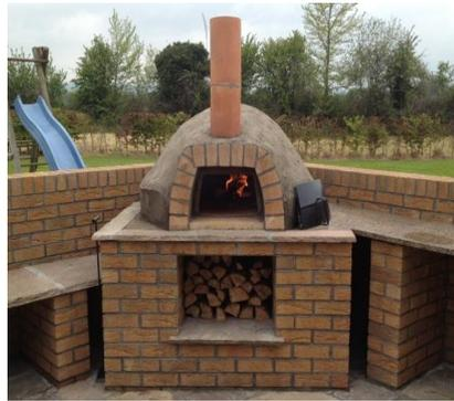
**Step 9:** Stick on slip bricks and add second flue if required.
