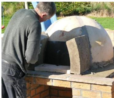
**Step 5:** Assemble the front arch as shown using modular arch bricks on each side. Insert the door to make sure it fits correctly before jointing the pieces.
